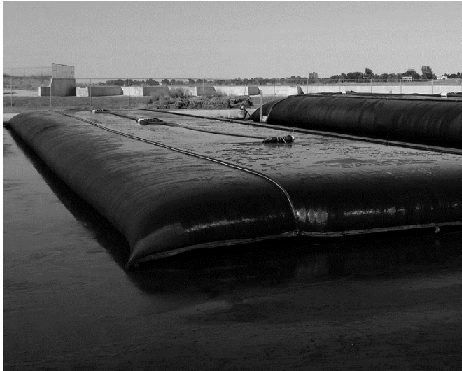
Fig 6. Geotextile dewatering tube
