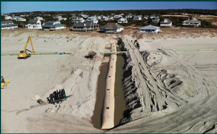
Geotextile Groyne Construction
