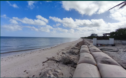
Beachfront Revetment Installation
