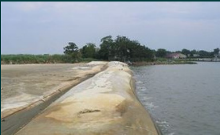
Perimeter Dyke for Marsh Protection
