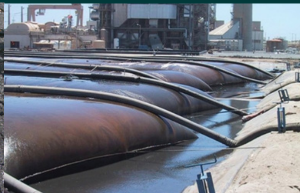
Geotextile tubes used for ash dewatering
