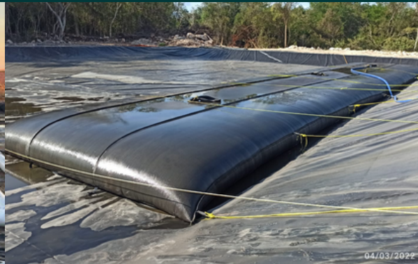
Titan tube technology applied for agricultural waste in a hog waste application
