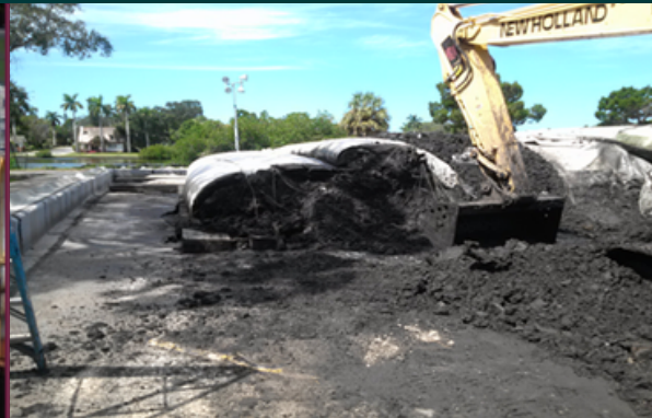
Dewatered sludge being removed from a Titan tube®
