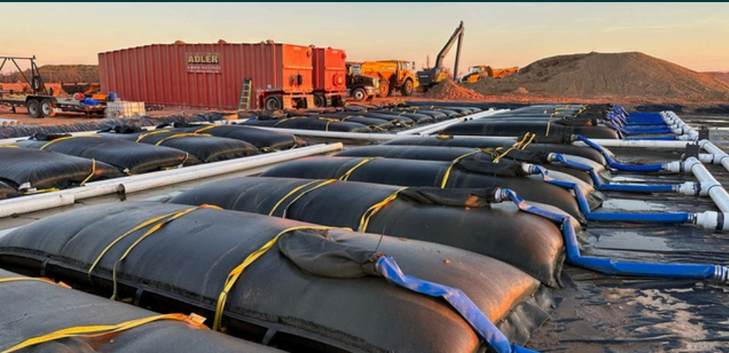
Titan tube technology applied for agricultural waste in a hog waste application
